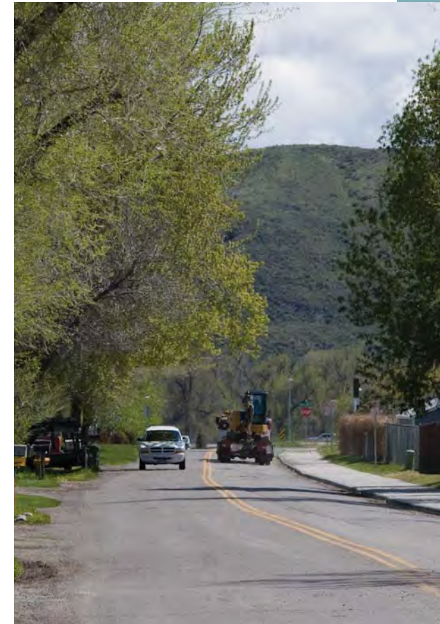
One capital improvement project recently completed was the installation of sidewalks on Jackson Street.
